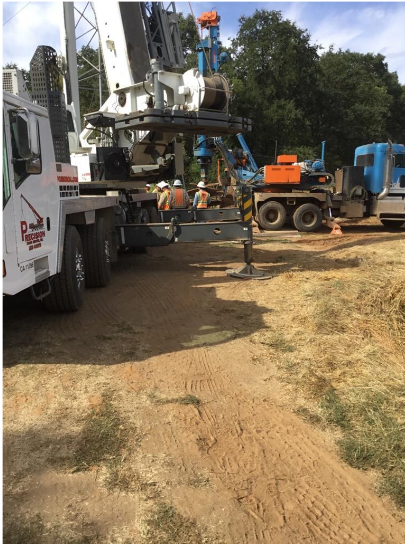
Photo 2: Drilling work for foundation installation at site 12/89.
